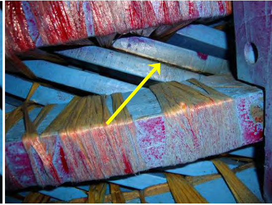
Figure 9: PD between Adjacent Phases
