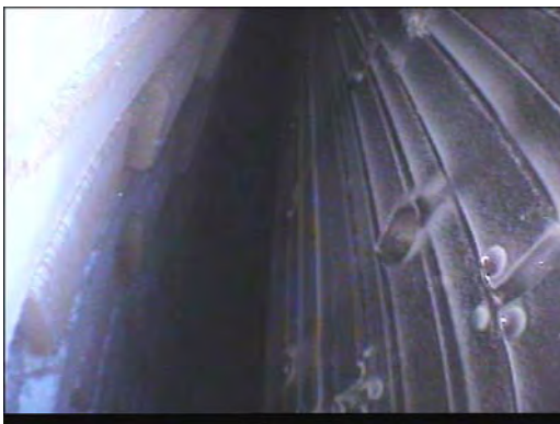
Figure 2: Drive End with Dirt and Oil
