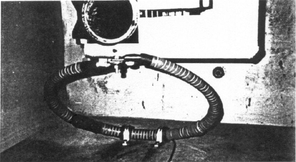
Figure 4 Photograph of a capacitive coupler installed on the generator bushing on one phase
