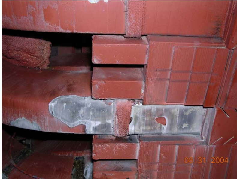
Figure 3: Deterioration at bar exits from core
