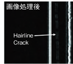
Post Imaging Processing Defect Image
