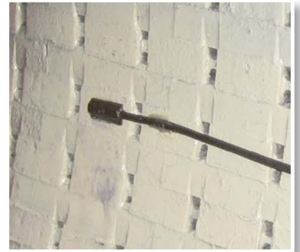
Iris Power TFProbe glued to a turbine generator stator tooth
