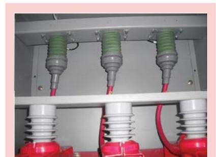
*Iris Power EMCs are sold in coupler kits complete with all installation materials including the silicone rubber insulating boot (EMC boot) shown here. Where required, insulating tapes are available.*
