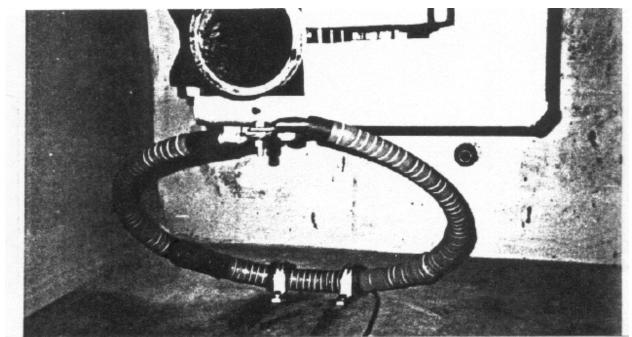
Figure 4 Photograph of a capacitive coupler installed on the generator bushing on one phase
