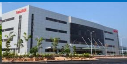
Integrated SSD / China backup facility
